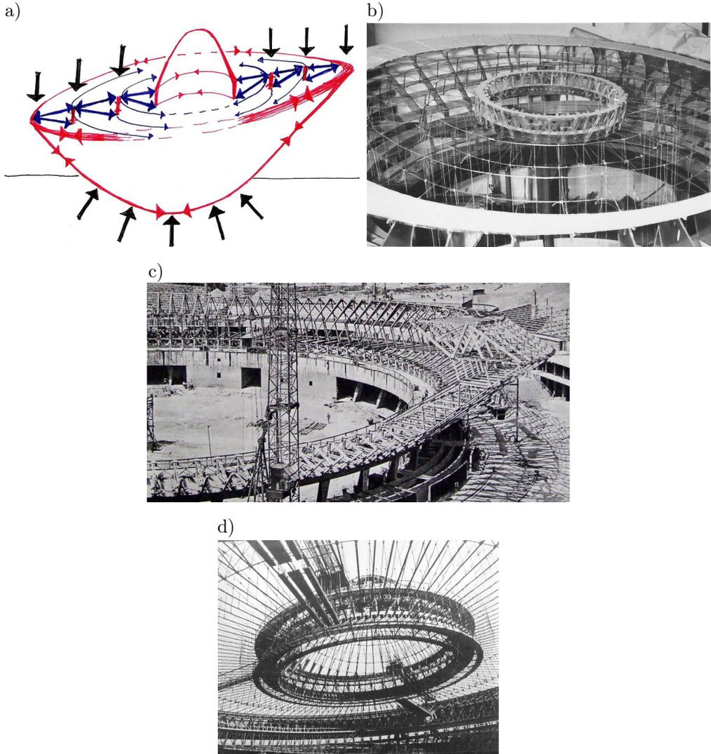
FIG. 12. a) Force diagram by E. Allen and D.M. Foxe (source: <http://www.wz-structure.org/#/spodek/>); b) scaled wired model used by W. Zalewski for structural concept testing (source: <https://structurae.net/en/structures/spodek>); c) external ring at the top of the bowl (source: <https://fotopolska.eu/195932,foto.html>); d) internal ring at the center of the roof suspended by tensioned cables (source: <https://structurae.net/en/structures/spodek>).
