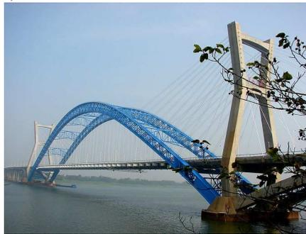
FIG. 13. Bridges combining cable-stayed and arch type of construction: a) Seri Saujana Bridge in Malaysia (source: [https://en.wikipedia.org/wiki/Seri\\_Saujana\\_Bridge#/media/File:Seri\\_Saujana\\_Bridge\\_2009.jpg](https://en.wikipedia.org/wiki/Seri_Saujana_Bridge#/media/File:Seri_Saujana_Bridge_2009.jpg)), b) Lianxiang Bridge in China (source: [https://commons.wikimedia.org/wiki/File:Lianxiang\\_bridge.jpg](https://commons.wikimedia.org/wiki/File:Lianxiang_bridge.jpg)).
