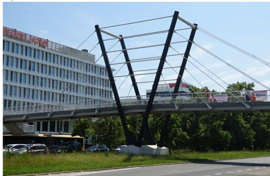
FIG. 14. Untypical bridges with double split-pylon: a) Flughafenbrücke near Düsseldorf airport (source: [https://commons.wikimedia.org/wiki/File:Flughafenbrücke\\_der\\_A44.jpg](https://commons.wikimedia.org/wiki/File:Flughafenbrücke_der_A44.jpg) ); b) footbridge in Warsaw (photograph by the first author).
